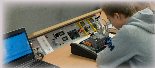
Power Distribution & Furniture for Lab
